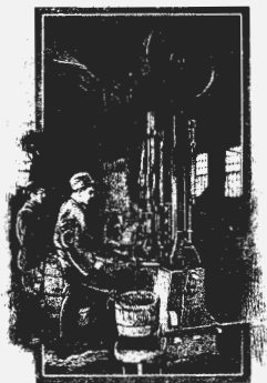
Welding the hard cutting edge to the tough frame
