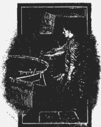
Hardening the Wiss Shear Blade
