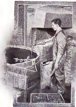
Hardening the Wiss Shear Blade
