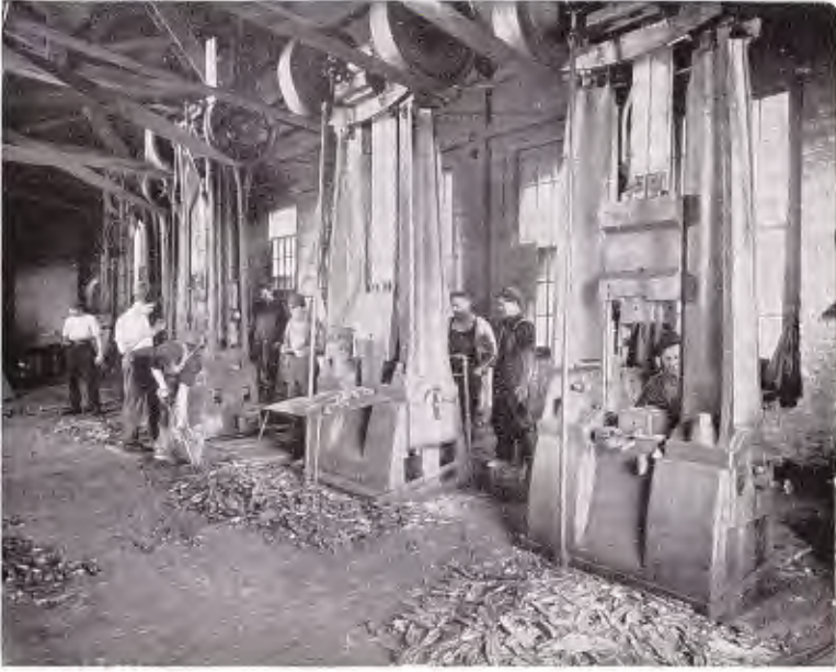
Wiss Forging Department where the frames of Wiss Shears are forged under powerful drop-hammers
