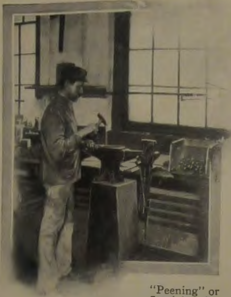
"Peening" or Straightening
