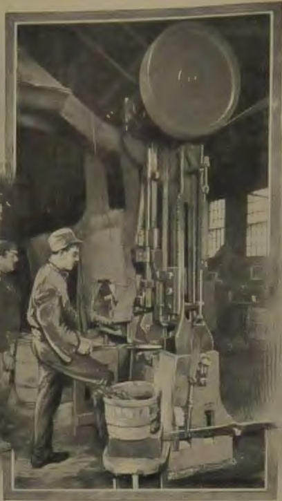
Welding the hard cutting edge to the tough frame
