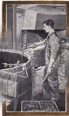
Hardening the Wiss Shear blade
