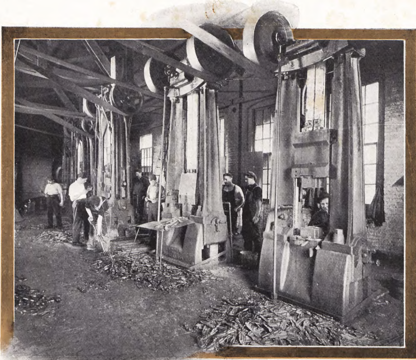
Wiss "Steelforging" Department where the frames of Wiss Shears are forged
